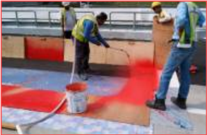
Painting of the Pit Lane Parc Fermé Using the Spray Method for the 2016 Shell Malaysia Motorcycle Grand Prix at Sepang International Circuit (SIC).
