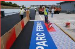
Painting of the Pit Lane Parc Fermé Using the Spray Method for the 2016 Shell Malaysia Motorcycle Grand Prix at Sepang International Circuit (SIC).
